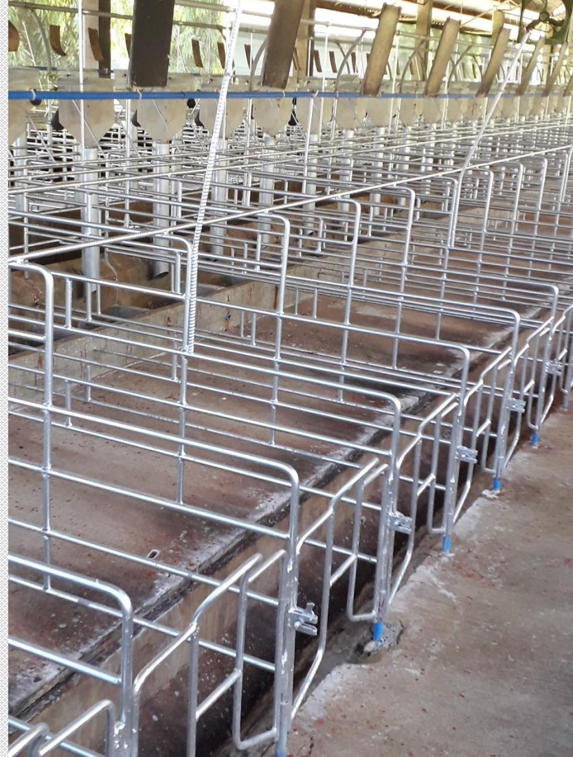
GESTATION PENS PAINTED
