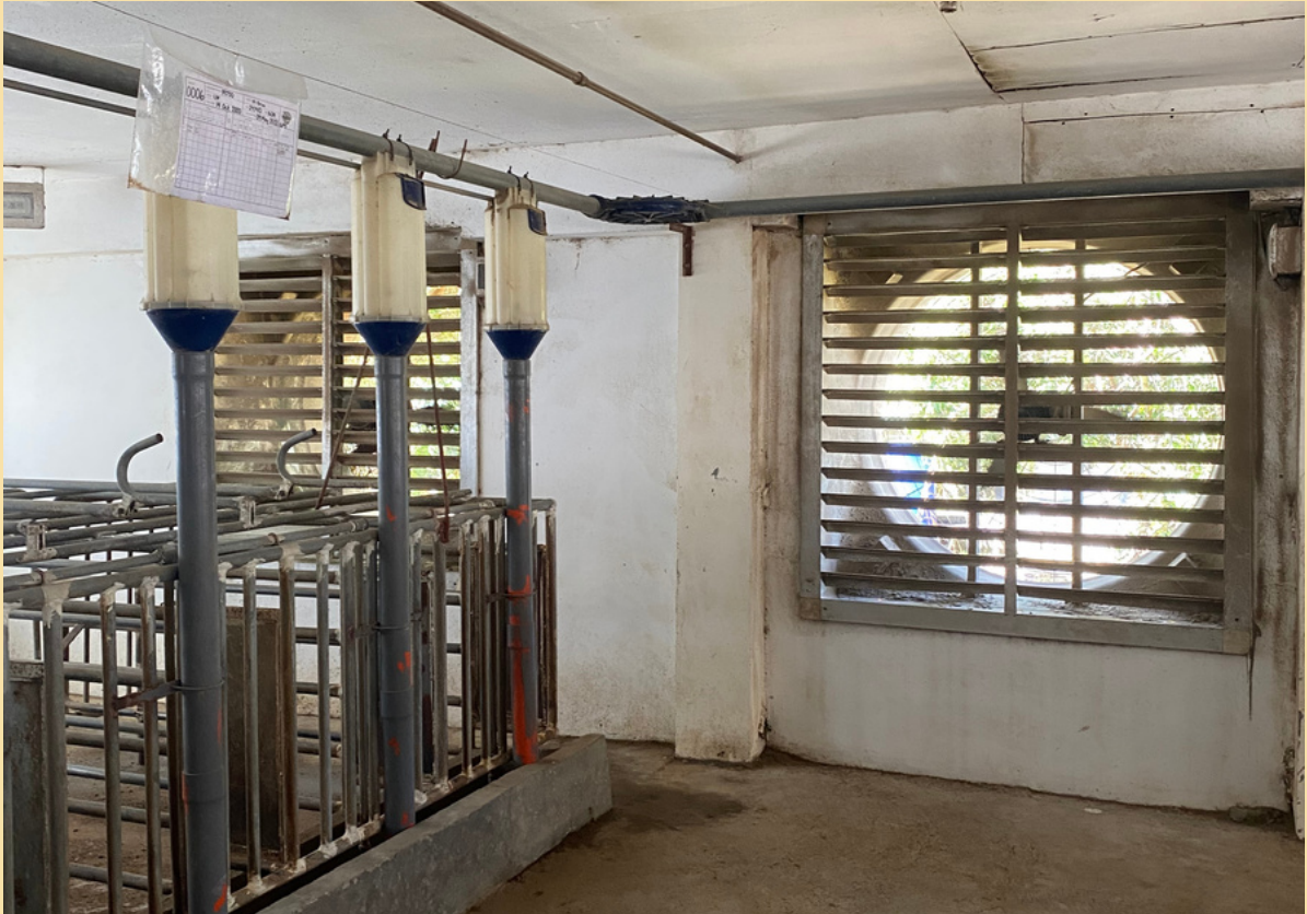
Image 10. Artificial ventilation using exhaust fan (Source: Photo taken at ATI-ITCPH, 2022)
