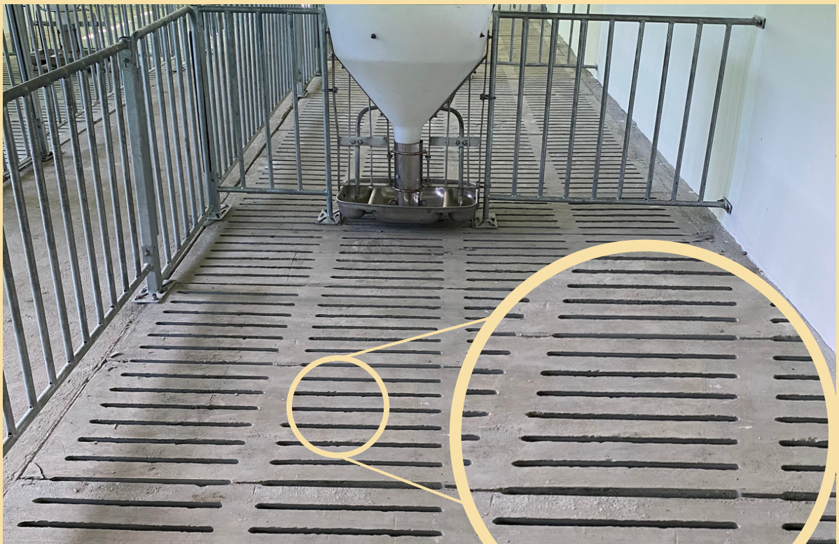
Image 18. Concrete flooring (Source: Photo taken at ATI-ITCPH, 2022)
