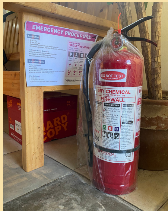
Image 29. Fire extinguisher (Source: Photo taken at ATI-ITCPH, 2022)
