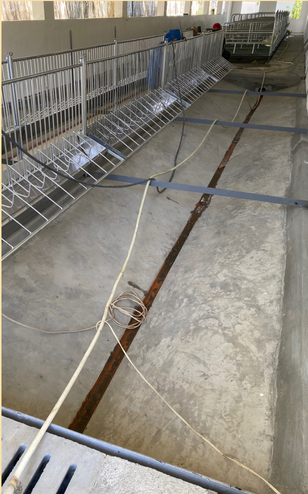
Image 48. Drainage system underneath the pens (Source: Photo taken at ATI-ITCPH, 2022)
